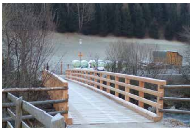
Wasserlechn-Brücke in Luttach
